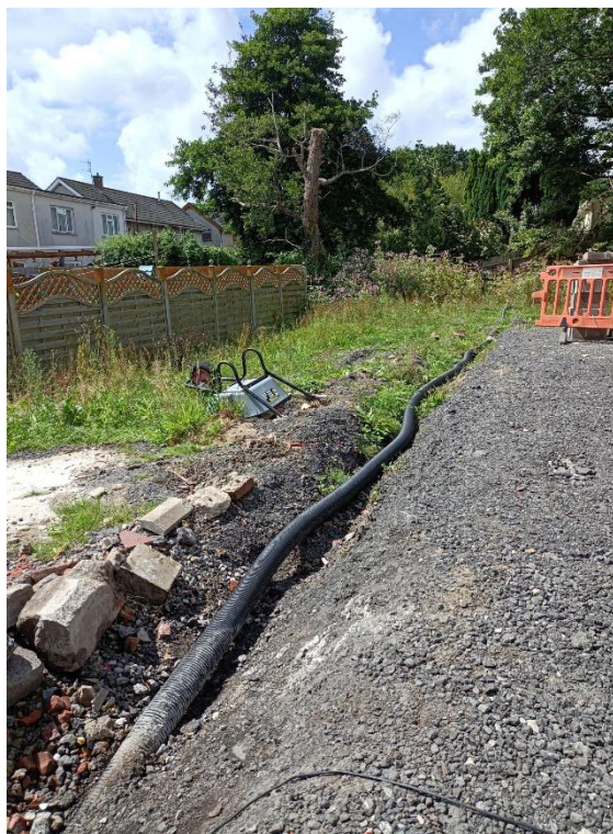
Fig. 5 - Looking towards the rear of the garden –
