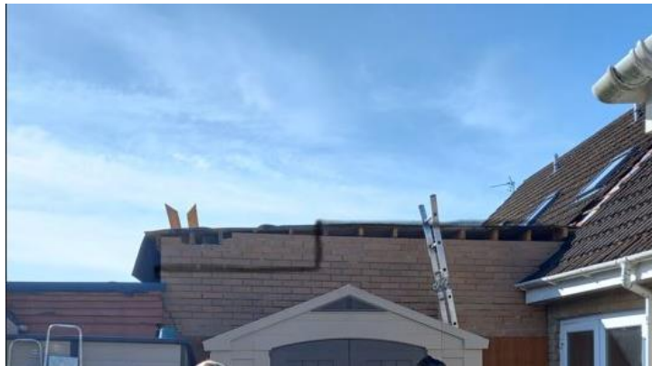
Fig. 6 – Relationship between the extension and 37, Hunters Ridge part way through construction
